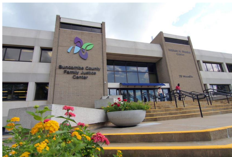
Buncombe County Family Justice Center. Photo courtesy of Buncombe County.
